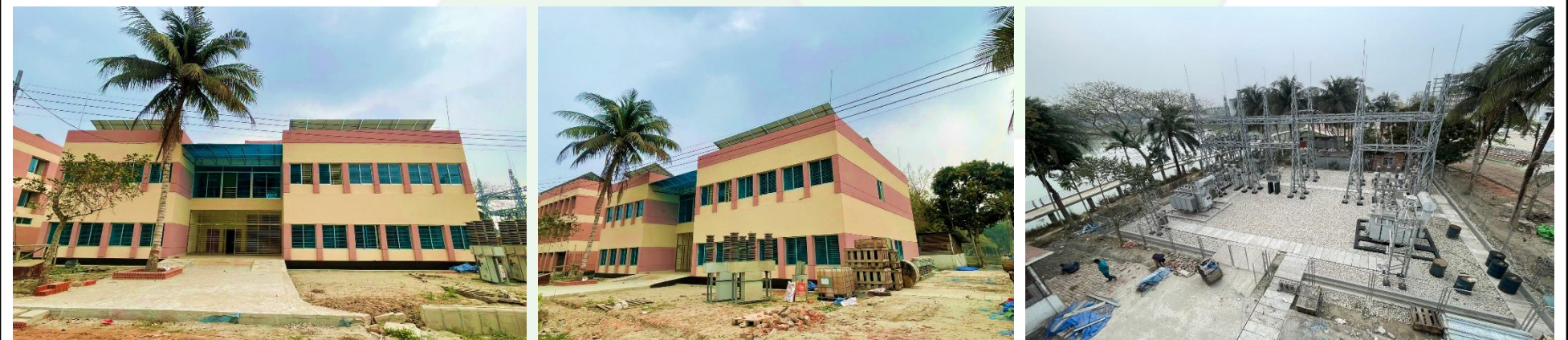
Name: 33/11 KV , 2*5/6.66 MVA Substation Location: Khulna University of Engineering & Technology (KUET), Customer: EnergyPac
