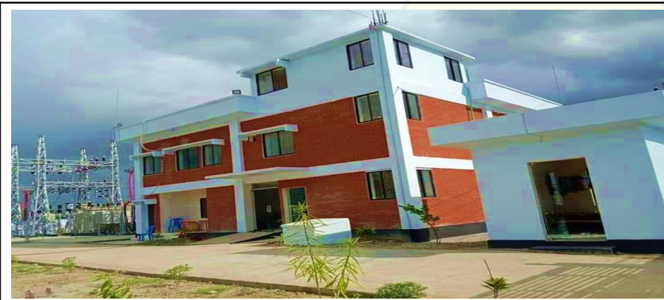
Name: 33/11 KV Sub-Station Location: Nagorpur-2 Customer: EnergyPac
