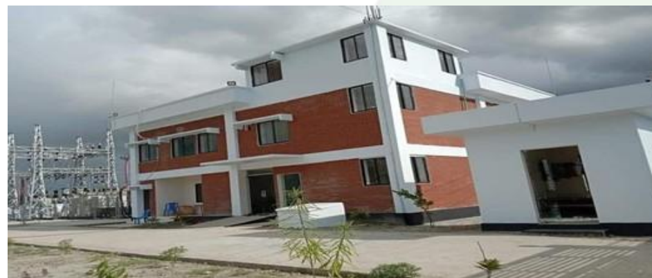
Name: 33/11 KV Sub-Station Location: Bhanga-3, Customer: EnergyPac
