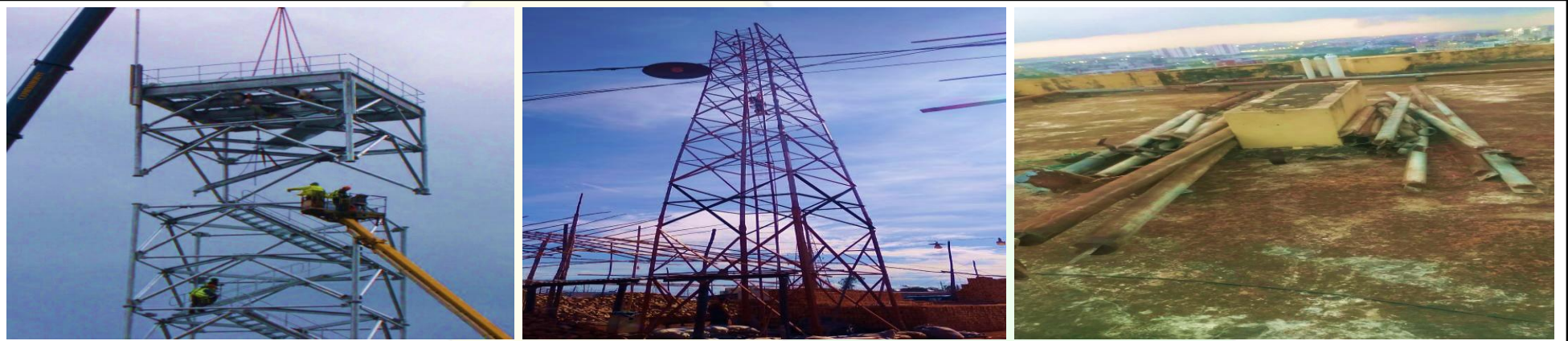
Name: Obsidian (Dismantle) Location: Barishal Customer: Edotco
