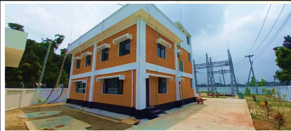
Name: 33/11 KV Sub-Station Location: Muradnagar-4 Customer: EnergyPac
