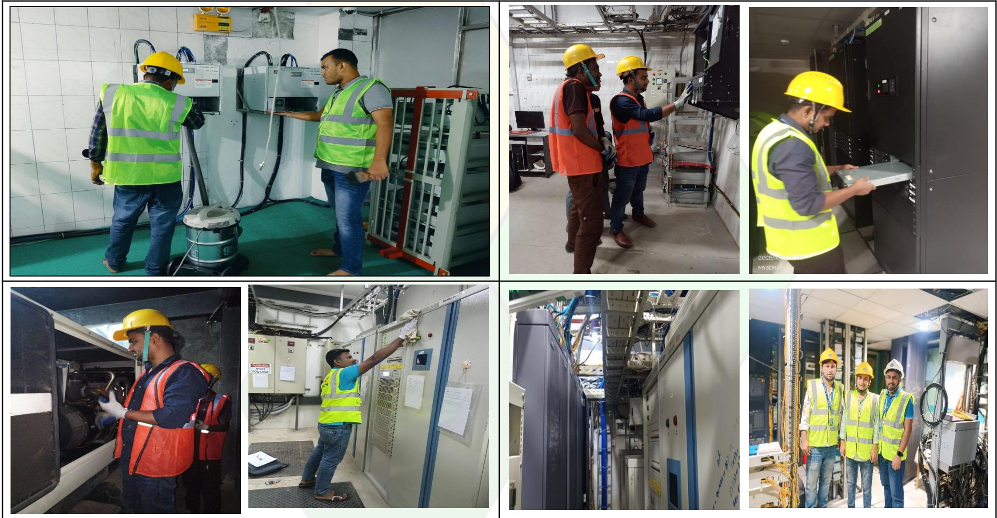
Sample Pictures of O&M Works
