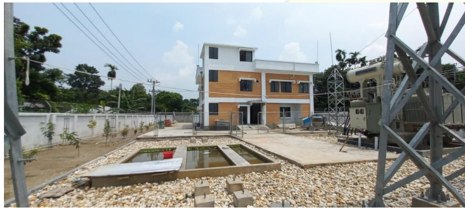
Name: 33/11 KV Sub-Station Location: Kalihati-4 Customer: EnergyPac
