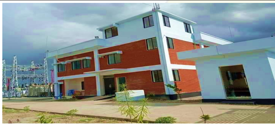
Name: 33/11 KV Sub-Station Location: Nagorpur-2 Customer: EnergyPac
