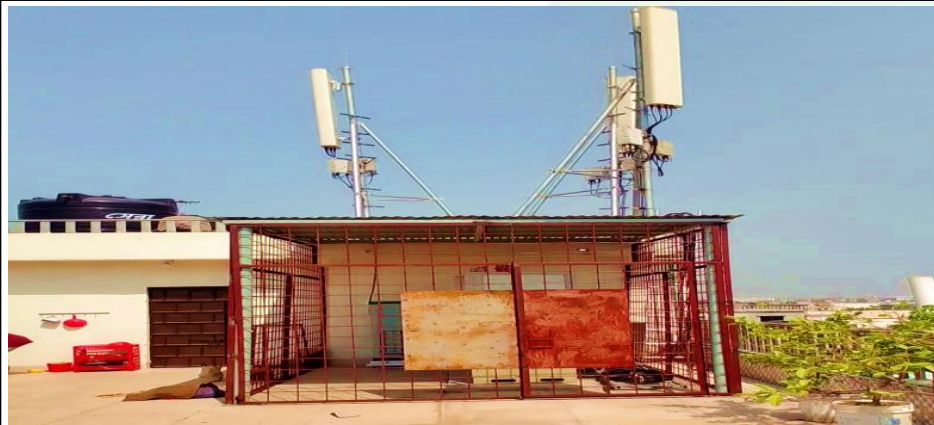
Name: Edotco Civil Project Location: Rangpur, Customer: Edotco (For Banglalink)
