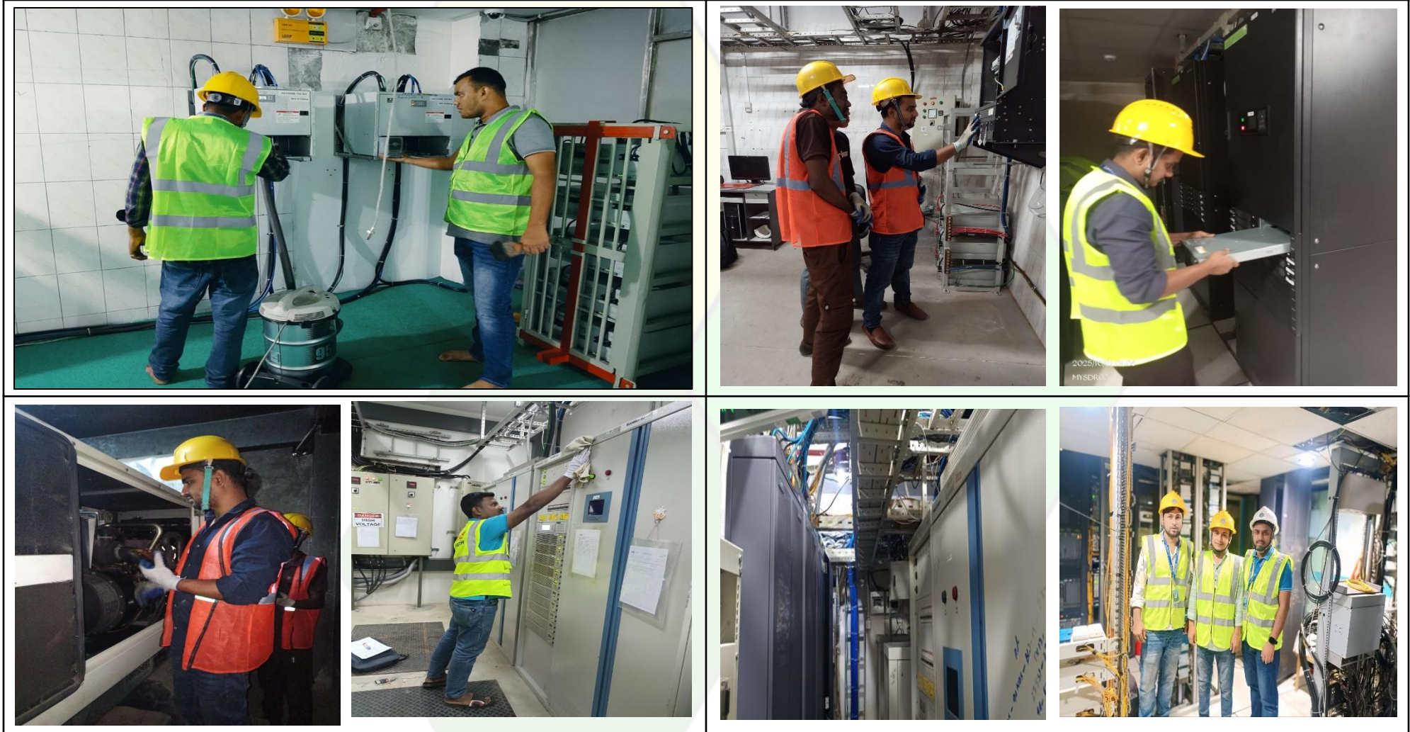
Sample Pictures of O&M Works
