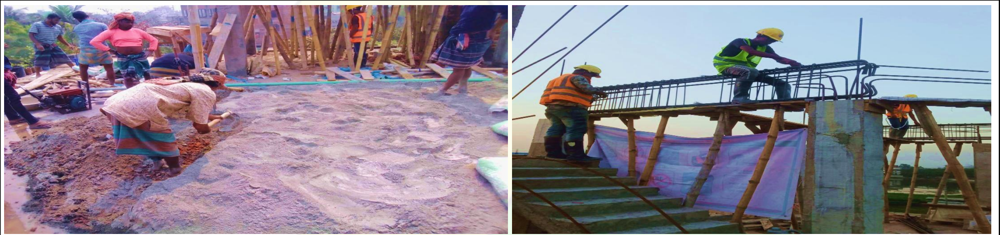
Name: Edotco Civil Project (NGHDRV4) Location: Narayanganj Sadar, Narayanganj Customer: Edotco
