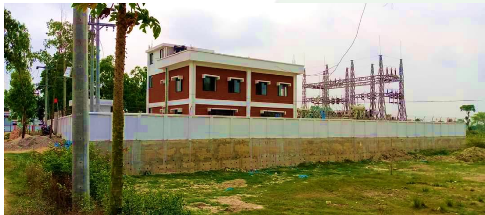
Name: 33/11 KV Sub-Station Location: Mirzapur-8, Customer: EnergyPac
